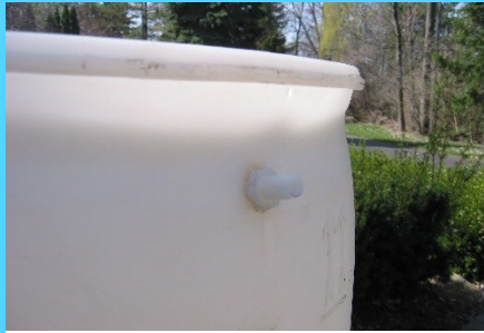
Upper hose barb for water overflow.
